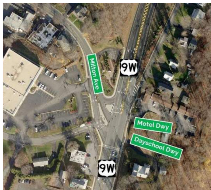
Exhibit 2 – US Route 9W and Milton Avenue/Dayschool Driveway/Motel Driveway
